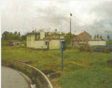
Anaerobic Sludge Digester
