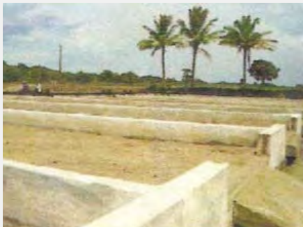
Sludge Drying Beds
