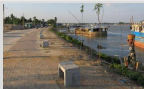
Fig. 9: Completed road segment with footpaths, street bench, and roadside drains.
