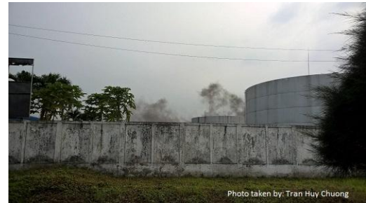
Fig. 4: Black smoke still observed from chimneys
