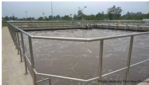
Fig. 2: Constructed WWTP in Tra Noc Industrial Zone
