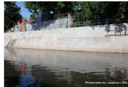
Fig. 13: Completed Segment of Flood Protection Wall
