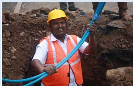
Fig. 12: Ongoing network improvement and pipe replacement works in line with 24x7 water supply PFS recommendations.
