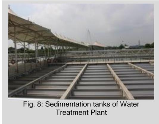
Fig. 8: Sedimentation tanks of Water Treatment Plant
