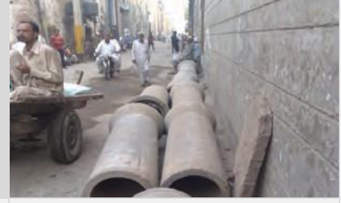
Improving the city's urban drainage system
