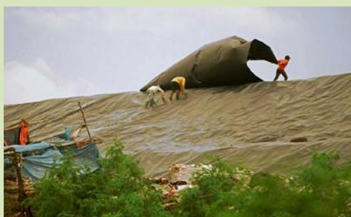
Fig. 15: Geo-membrane technology currently in use at the Rawa Kuching landfill site.
