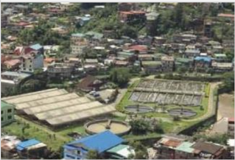
Baguio Sewerage Treatment Plant (BSTP)
