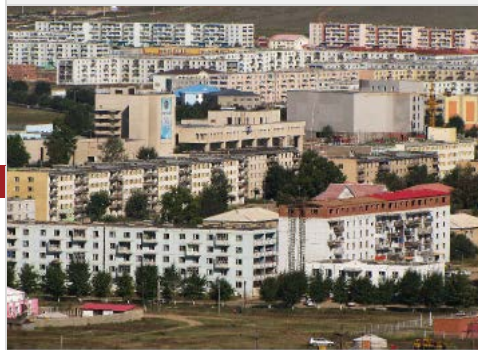
Typical apartment buildings in Darkhan
