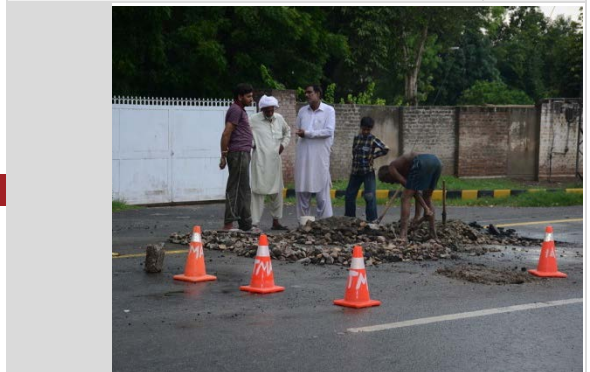
On-going repair work on water source
