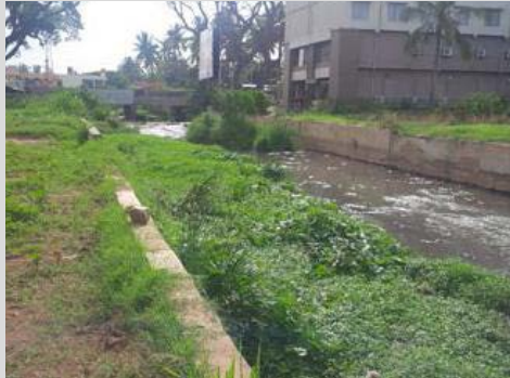
Lower concert drain walls constructed adjacent to the hospital
