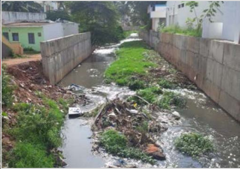
Construction of high concrete drain walls
