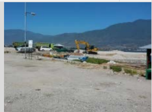
Reclamation near Swiss Belhotel
