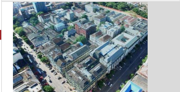
Aerial view of Pansodan Cluster
